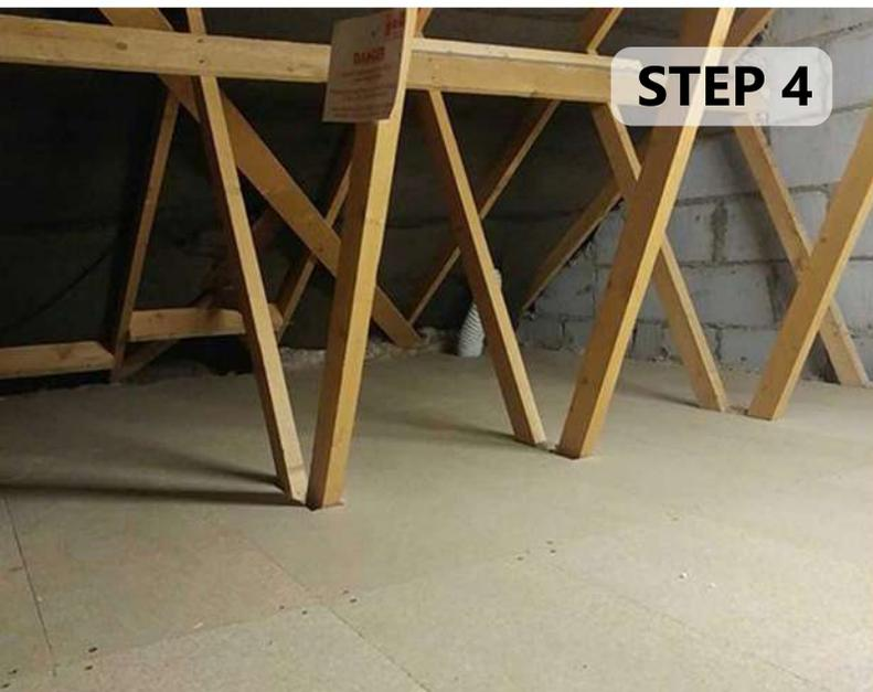
You can now board over with tongue and groove Loft Boards (1200mm x 325mm) or floor grade boards (600mm x 2400mm) to create a usable space for storage.
