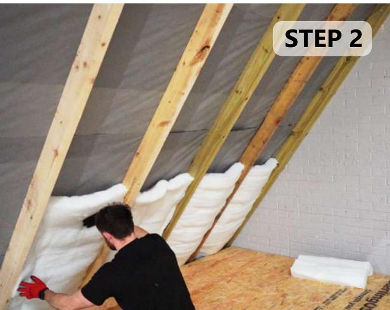
Install your EcoLoft Non-Itch between rafters, by rolling the material out between. You can cut the EcoLoft Non-Itch at the end of a run with our Multifoil Insulation Scissors to remove any excess, which can then be used to start your next run.
