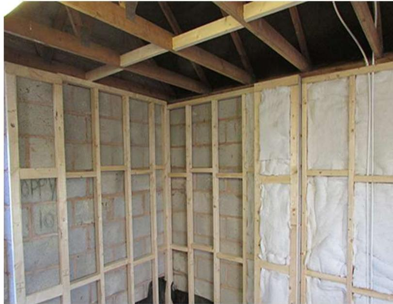
Place the EcoLoft Non-Itch between the studwork. If any part of your wall is at an angle, you can make the necessary cuts to ensure this slots neatly in place. You can then board over. For improved performance you can install a layer of our EcoQuilt Expert, before installing a 25mm batten and plasterboard.
