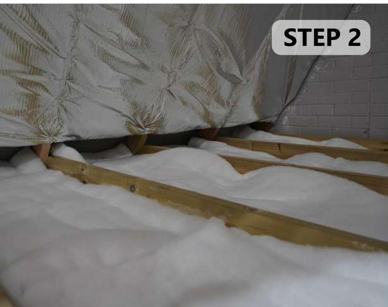
Roll out the EcoLoft Non-Itch and install between the floor joists. You can cut the EcoLoft Non-Itch at the end of a run with our Multifoil Insulation Scissors to remove any excess, which can then be used to start your next run.
